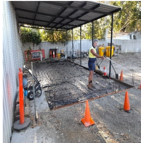
Jim Whatley prepped the area for the arrival of the concrete
